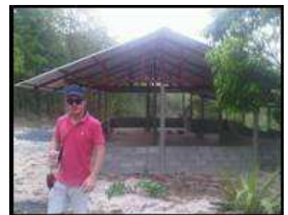
Lahu Orphanage being built →
